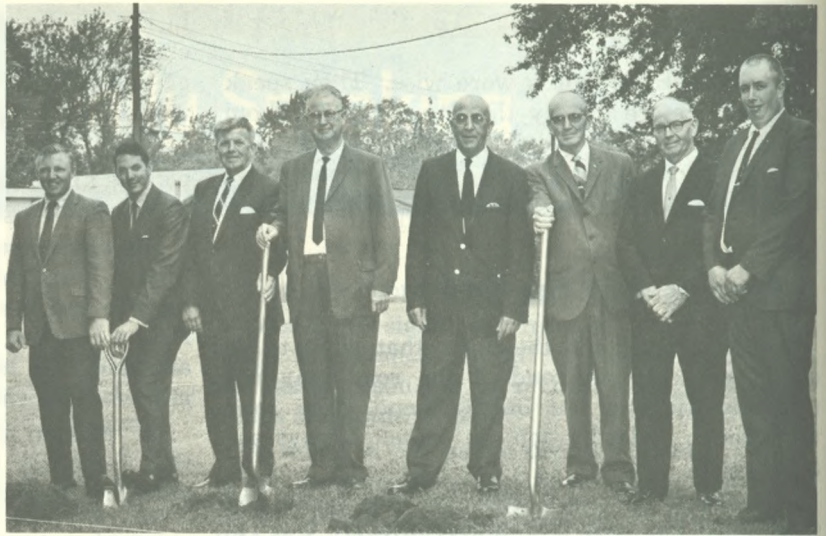
THE TRUSTEES and members of the building committee of the St. Bernice (Ind.) First Church take their turn at a ground-breaking service for a new educational building at the church site. The brick-and-block building is scheduled for completion in mid-January, 1970. Rev. Claude D. Wilson is the pastor. Pictured from left to right are: Maurice Shaw, Sunday school superintendent; Ron McDonald, secretary of the board; Chancy Lewis, trustee; J. Les Maloney, trustee; Ted Plank, trustee; Warren Ferguson, trustee; T. R. Endicott, chairman of the board of trustees; and Ted Gordon, member of the building committee.
